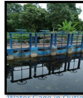
Water Gage in Outlet
