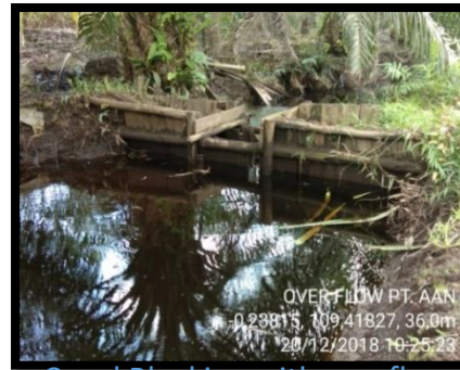
Canal Blocking with overflow
